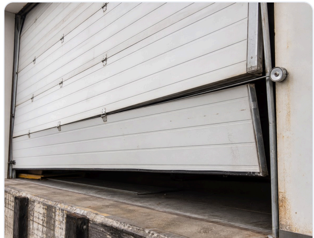
Loading dock door #3 — Door off its track; re-tracked and roller replaced.
