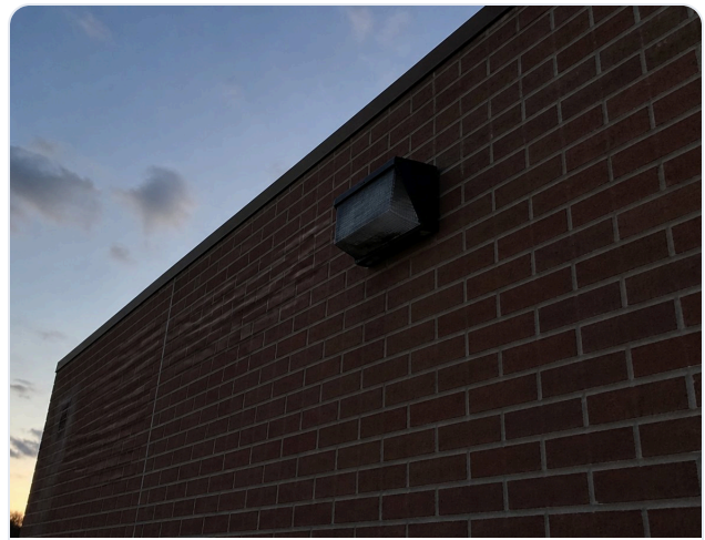
Exterior wall-pack (east) — Fixture out; replaced with LED.
